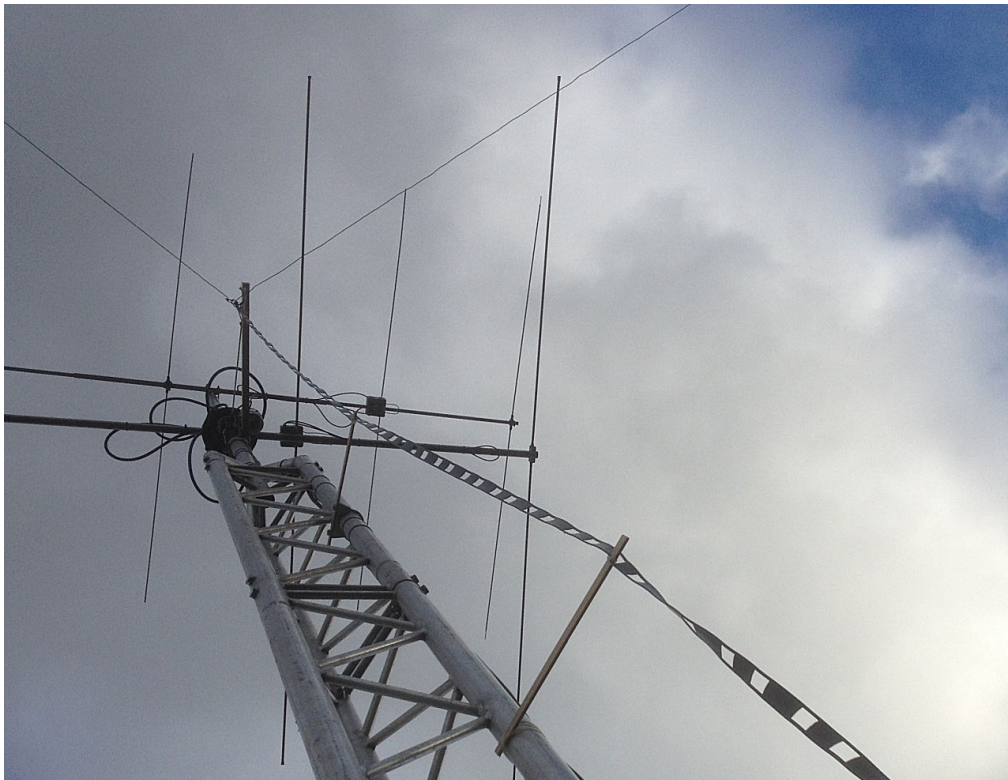
My balanced feeder system - wooden supports keep the ladder line away from the tower
